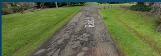
Unsealed Road with Dust Suppression Seal
