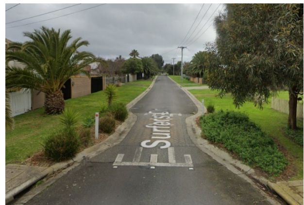
Single lane speed hump – Surfers Drive, Cape Woolamai
