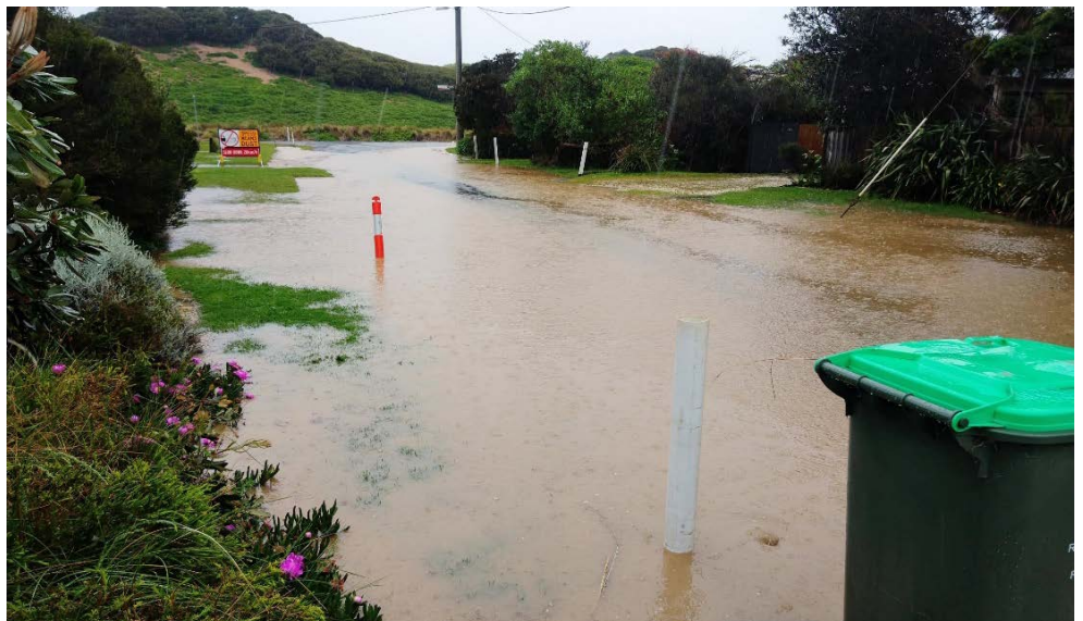
Glen Street after heavy rains this month
