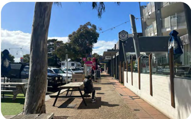
The built form and retail frontages on Marine Parade are a patchwork of styles and heights.
