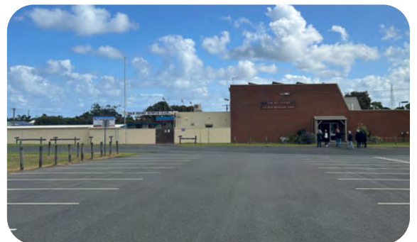
The Recreation Centre could be renovated or redeveloped to better cope with the demands of future growth
