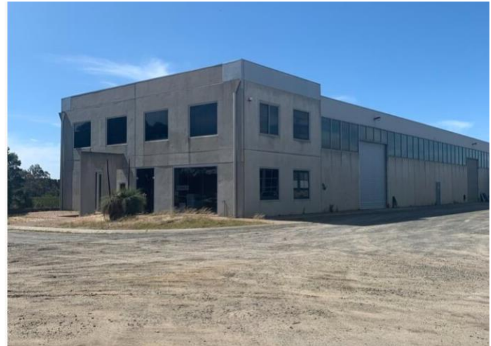
Figure 4-2: Example of Unsealed Accessway in Industrial Precinct
